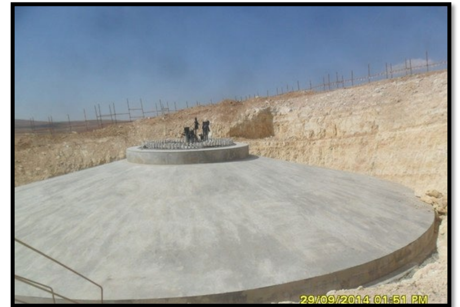
Completed Foundation ready for backfilling
