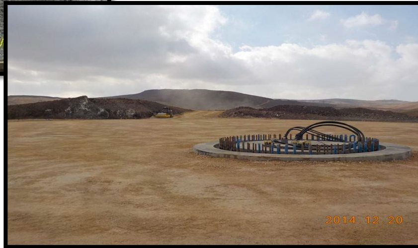
Backfilled Foundation
