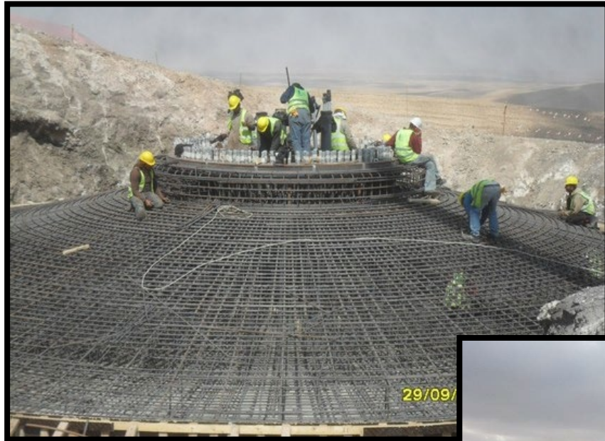
Foundation Reinforcement works
